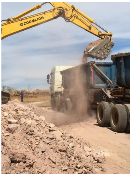
Figure 2. Trucks being loaded with ore
