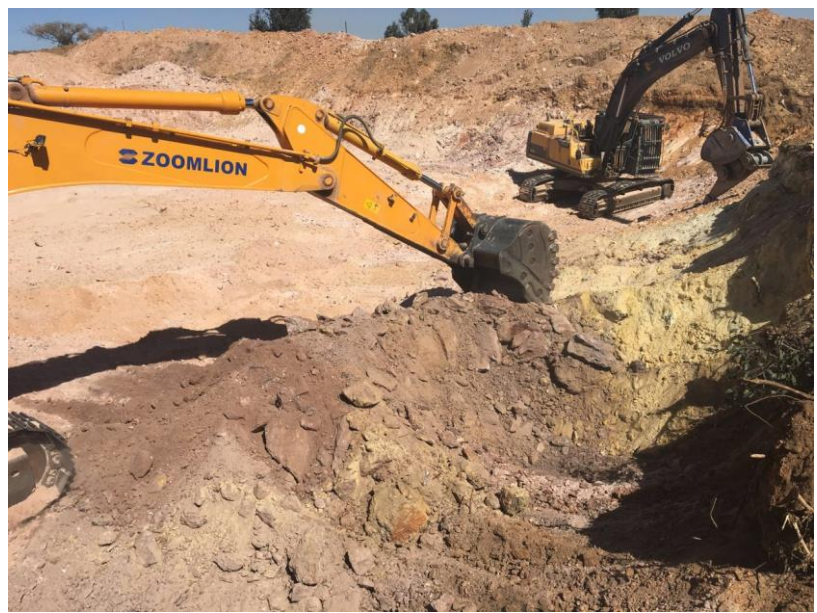
Figure 3. Ore being ripped and prepared for removal
